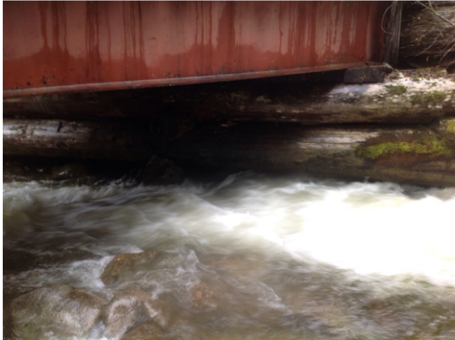
Right Bank Abutment when facing downstream
