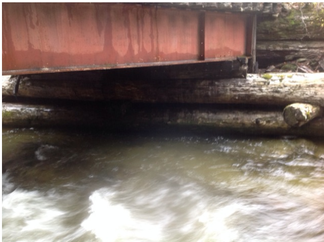
Left Bank Abutment when facing downstream
